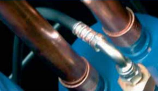
For centralized refrigeration installations with several compressors working in parallel, oil return is sometimes difficult to control completely, especially when the suction-gas velocity goes below a certain value, which is influenced by the pipes design (diameter & special configuration, vertical or horizontal). The same constraint is found on installations using compressors with variable-speed control.
