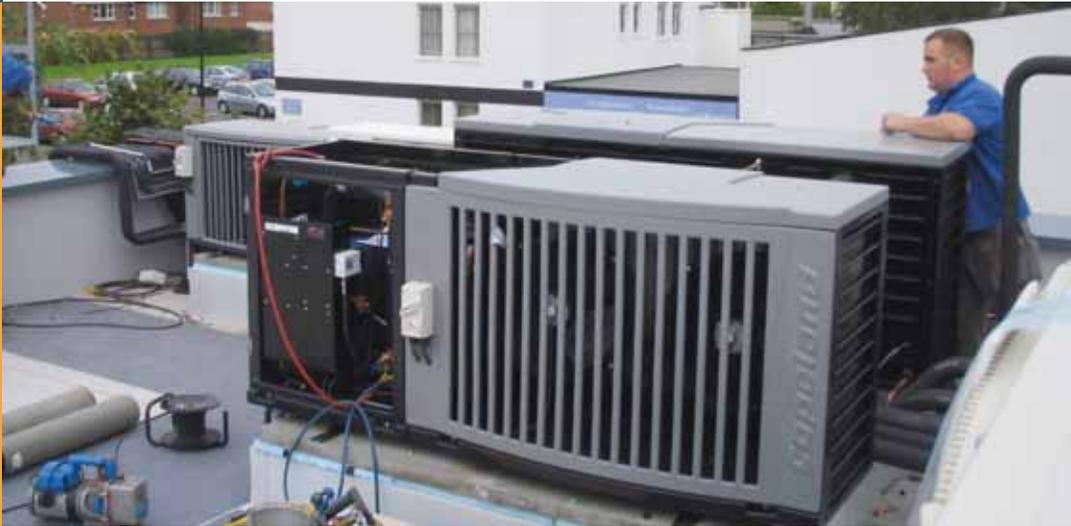
A Copeland Eazycool™ Network has a built-in oil management system. Each condensing unit has its own Alco Controls oil separator, thus limiting the transfer of oil to the system, and each compressor is fitted with a Traxoil electronic level control. The distribution of oil between the units is achieved by a set of piping connected to the oil outlet and return valves on each installed unit. An oil reservoir is also provided within the Master unit.
